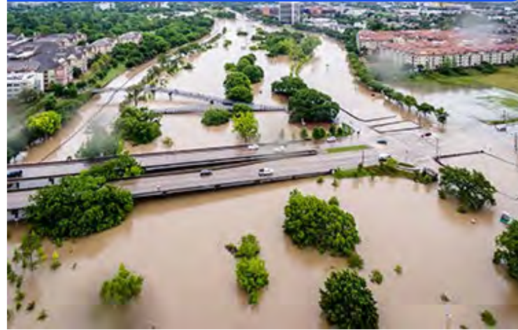
Tax Day Flood (2016) 9,820 structures flooded, 7 deaths
